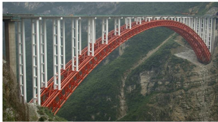
Fig 4. Typical CFST arch bridge
