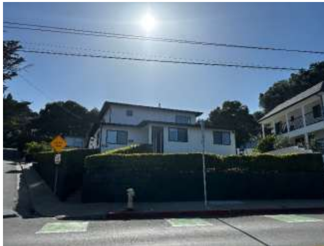
Figure 2. Example Low-Risk home (Neighborhood 5). Visible features include Class A roofing, stucco siding, double-pane windows with metal frames, maintained defensible space, and no vegetation contact with the structure.
