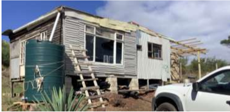
Figure 2. Incremental House Construction in an Informal Settlement, Cape Town (Source: authors)
