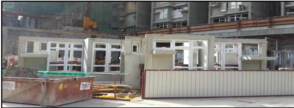
Figure 2: Company D site in Hong Kong for Precast construction
